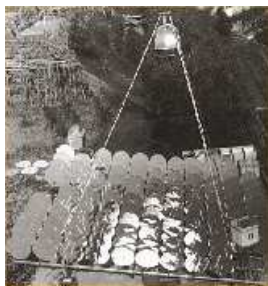
Fig. 3 – Point focus Fresnel reflector first system, Sant'Ilario Station, 1965 (Francia Archive)
