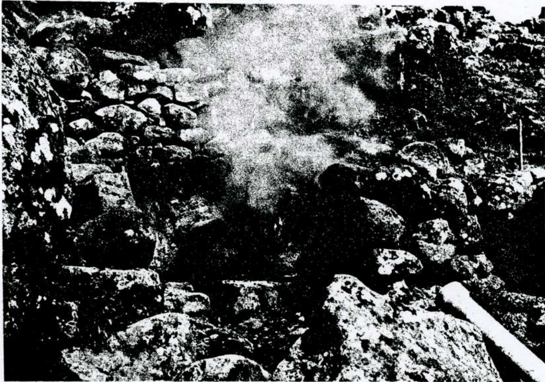
Figure 3. One of the steam sources is closed. The emerging tube will be connected with the condensation system.
